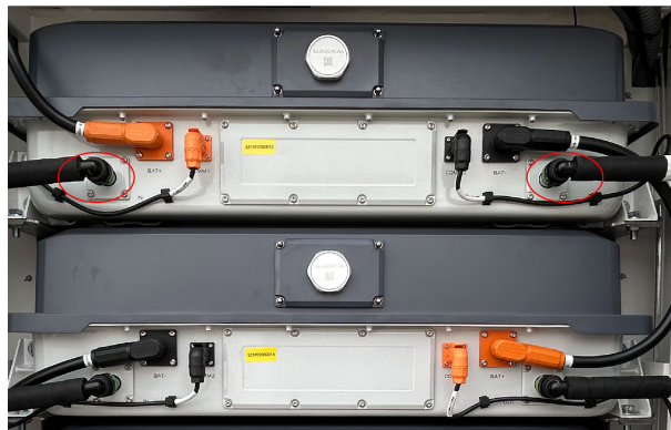
Figure 5-7 Positions of Liquid Cooling Pipes
