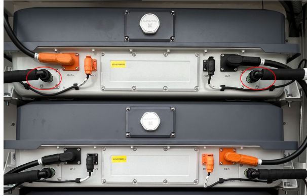
Figure 5-14 Positions of Liquid Cooling Pipe Fittings
