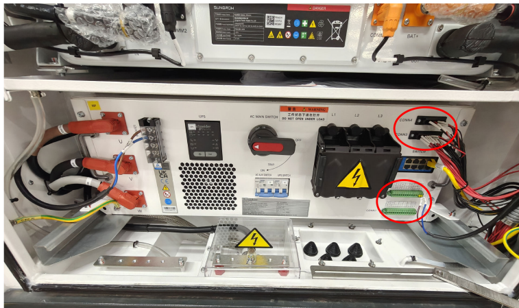
Figure 5-18 Position of CONN1–CONN4 Terminals
