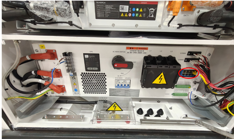
Figure 5-17 Position of Network Port
