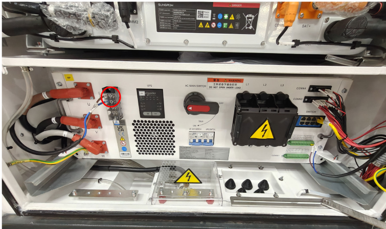
Figure 5-16 Position of Power Supply Cable
