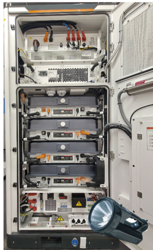
Figure 3-15 Inspect with Flashlight or Searchlight
