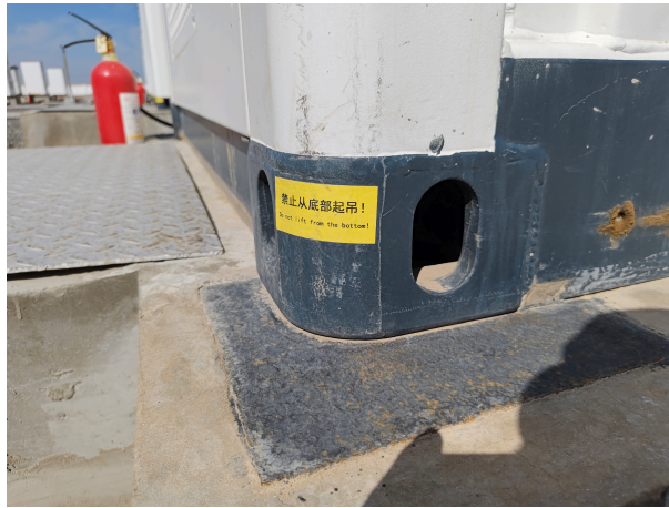
Figure 3-2 Secured by Welding
