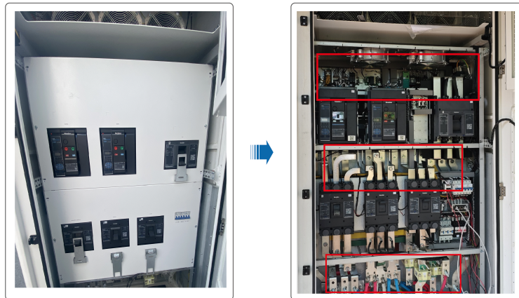
Figure 7-11 Locations of Screws
