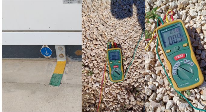
Figure 7-22 Measure Resistance at Grounding Point
