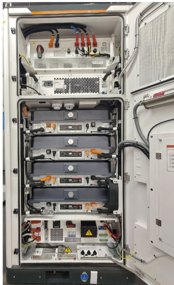
Figure 3-17 ESS Cabinet Interior
