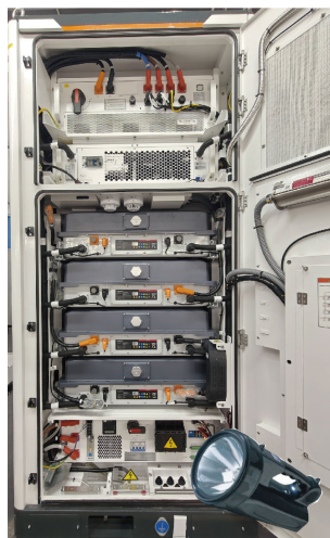
Figure 3-14 Inspect with Flashlight or Searchlight
