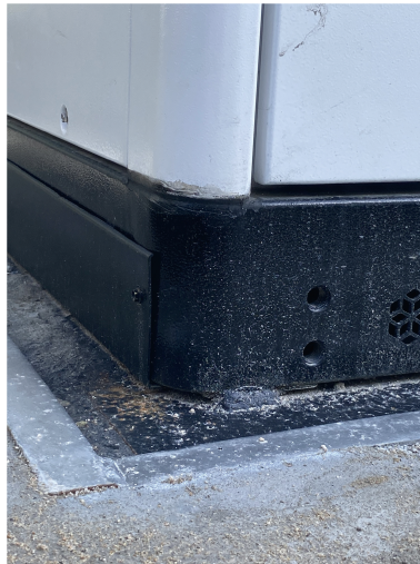
Figure 7-2 Secured by Welding
