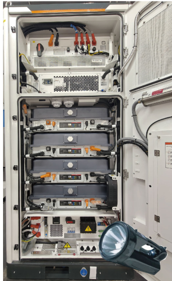
Figure 3-32 Inspect with Flashlight or Searchlight
