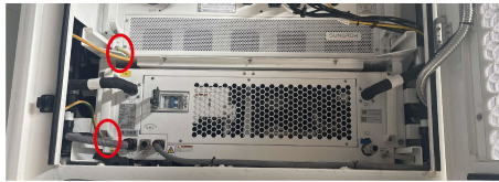
Figure 3-28 Equipotential Bonding Connections
