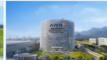
Yiwu Global Photovoltaic Joint Innovation Center
