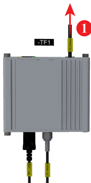
Figure 4.14 Removing power cable from 4G router
