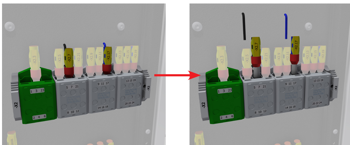
Figure 4.3 Splitting the cables
